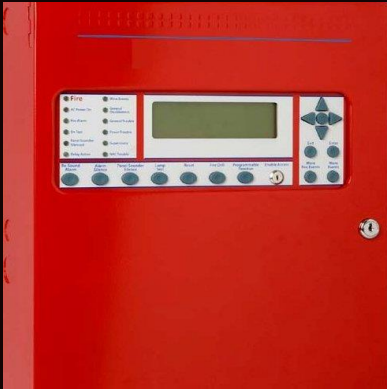
Fire Alarm Control Panel
