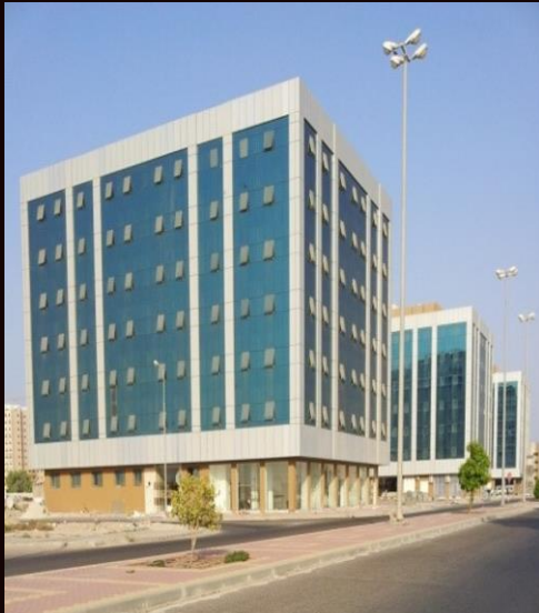
Shiekh Marawan 3 Buildings
